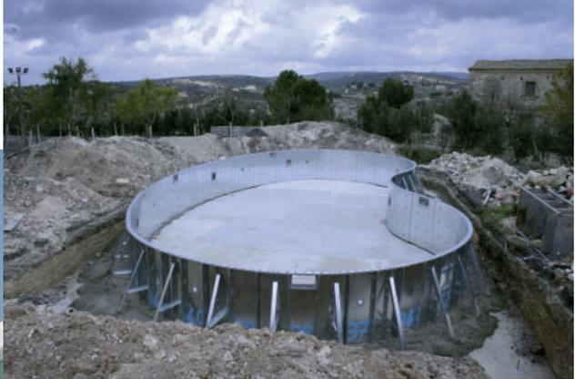
We can build structures for swimming pools of any type, underground or above ground, for gardens, for wellness centers or Olympic swimming pools. Our panels replace the concrete structure, making installation much easier, saving time and money.
